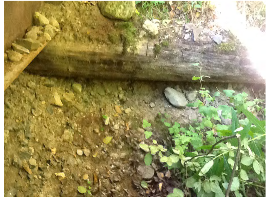
Right Bank Abutment when facing downstream
