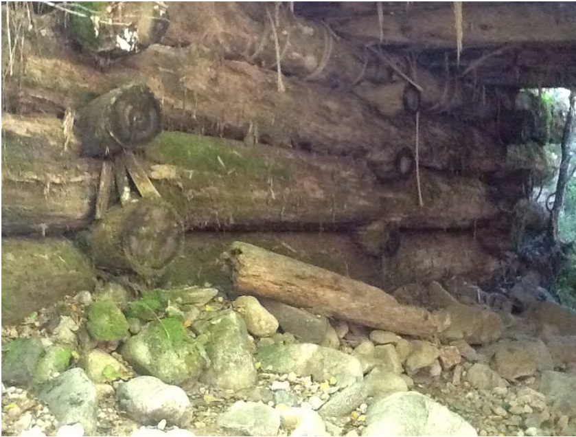
Left Bank Abutment when facing downstream
